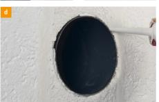
Seal the wall duct to the masonry inside and outside with a suitable sealing compound.
