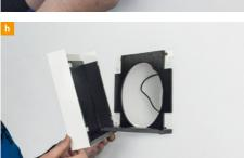
Connect the plug-in connection of the connection cable to the **AIRUNIT** control 2.0.
