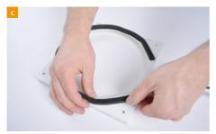
Stick the supplied sealing tape all around the back of the outer wall bracket.
