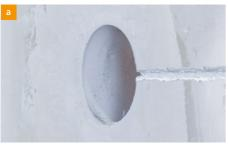
Make a core hole with a diameter of 162 mm.
