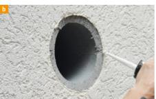
After completing the insulation / plastering work, remove the plaster covers on the inside and outside. Adjust the wall duct to the dimension of the finished wall by shortening the wall duct flush with the wall on the room and facade side using a carpet knife or hot wire.
