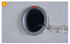
Insert the connection cable (min. 2x2x0.6 mm) into the wall bushing.
