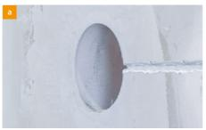
Make a core hole with a diameter of 200 mm.
