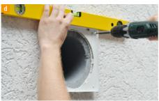
Mount the wall bracket of the weather protection bonnet with suitable fastening elements.
