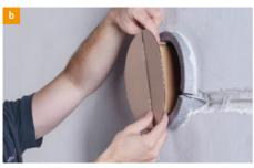
Close the wall duct on the inside and outside with the supplied plaster covers to prevent soiling of the wall duct.
